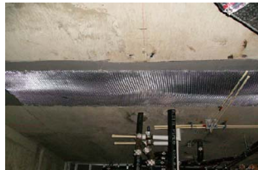
Figure 24 Fire proofed CRFP panel on underside of
