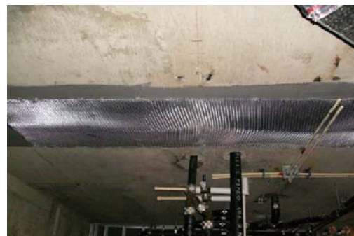
Figure 30 Installed CFRP with 2 hour fire proofing
