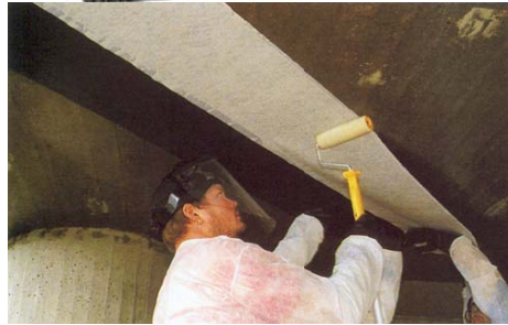
Figure 27 A roll of CFRP (top), CFRP installation (bottom)
