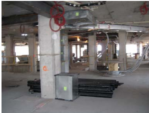
Figure 28 Typical installed material requiring
