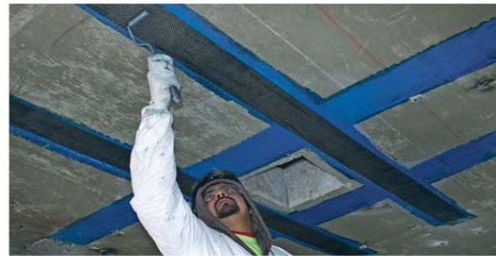
Figure 29 Installation of CFRP
